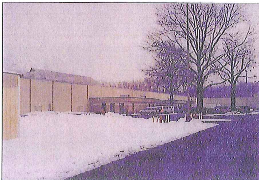
EAST ELEVATION OF INDUSTRIAL BUILDING WITH NEWER OFFICE ADDITION
