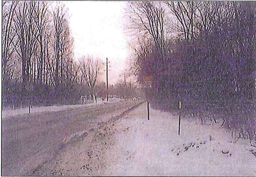
STREET SCENE LOOKING SOUTH ON WOODLAND AVENUE
