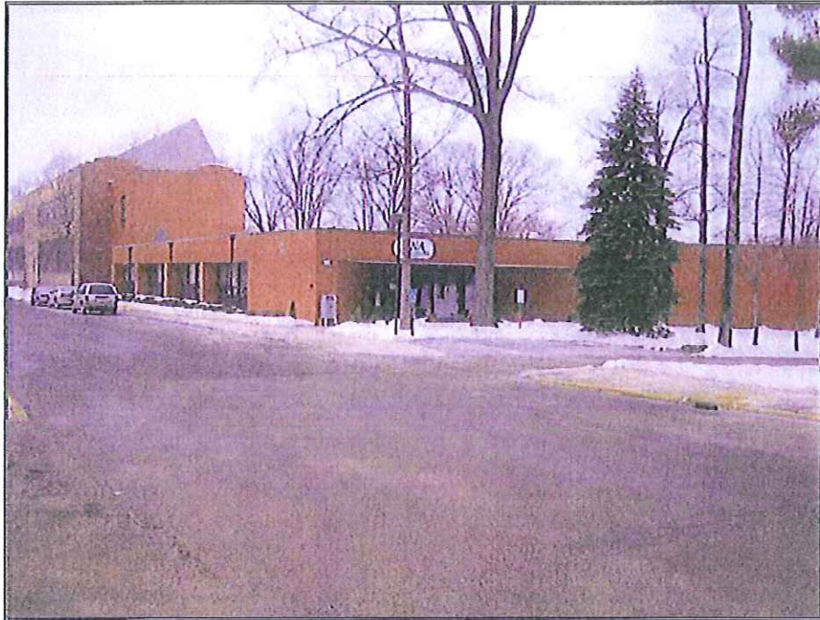
SUBJECT PROPERTY - NORTHERN (OFFICE) BUILDING
