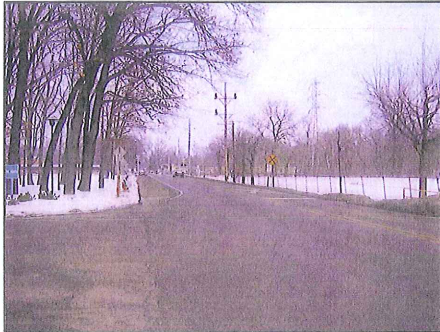
STREET VIEW - LOOKING NORTH ALONG WOODLAND AVENUE
