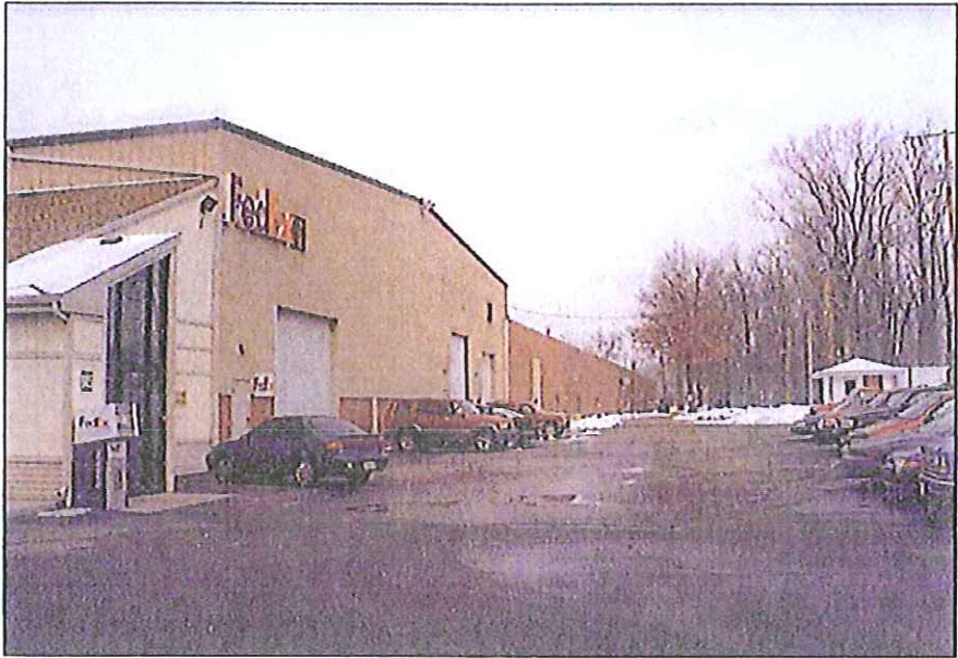
EAST ELEVATION OF INDUSTRIAL BUILDING (FRONT)
