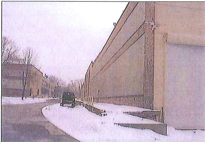
NORTH ELEVATION OF INDUSTRIAL BUILDING
