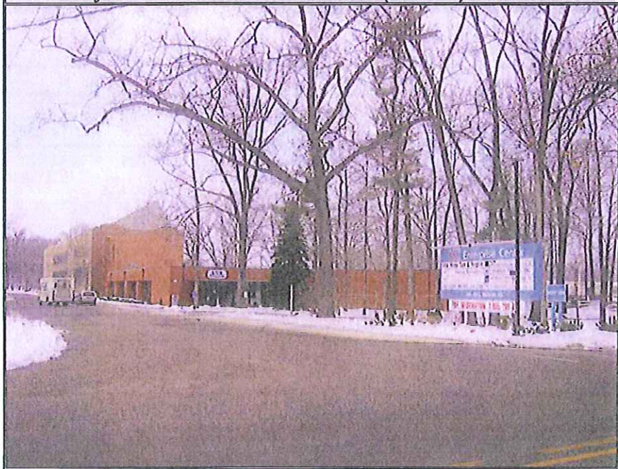
SUBJECT PROPERTY - NORTHERN (OFFICE) BUILDING
