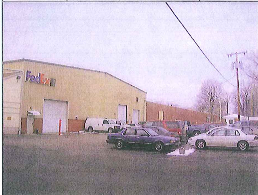
SUBJECT PROPERTY - SOUTHERN (WAREHOUSE/LIGHT INDUSTRIAL) BUILDING
