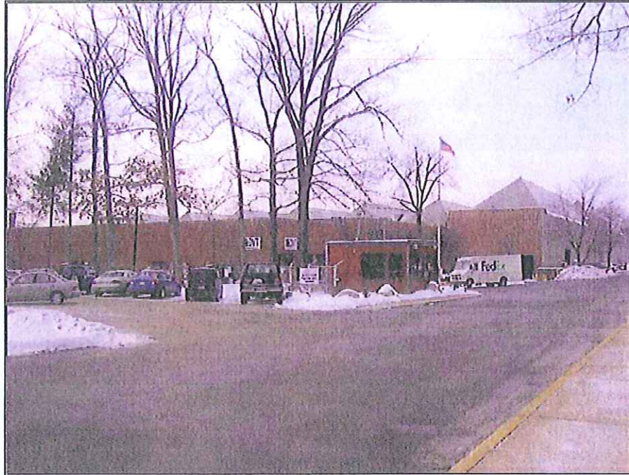
SUBJECT PROPERTY - SOUTHERN (WAREHOUSE/LIGHT INDUSTRIAL) BUILDING
