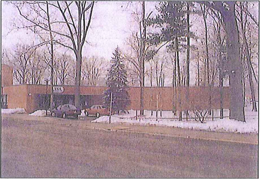
EAST ELEVATION OF OFFICE BUILDING (FRONT)
